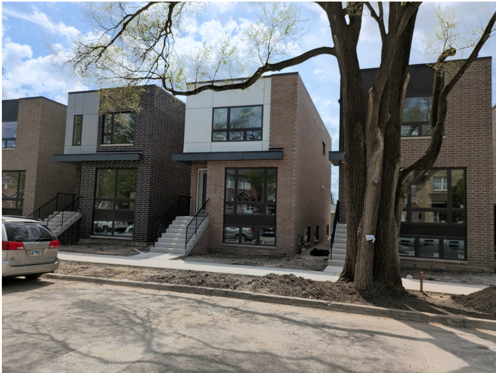
New construction - 2520 S. Stark (center house) Photo Credit: Michael E. Byczek. Copyright 2026.
