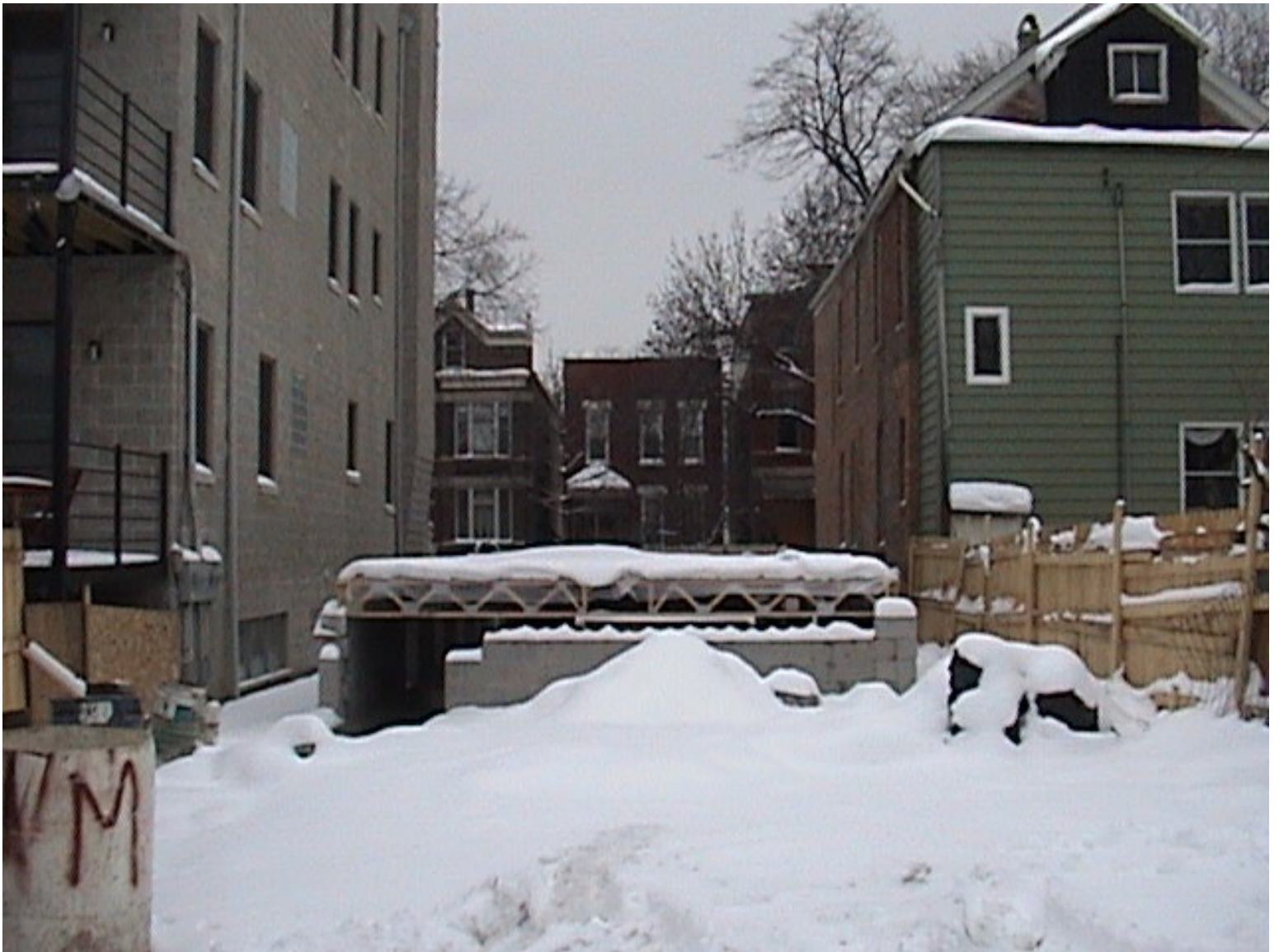
946 N. Winchester New Construction (View from Alley looking towards Winchester) Photo Credit/Copyright: Michael E. Byczek. About 2005.
