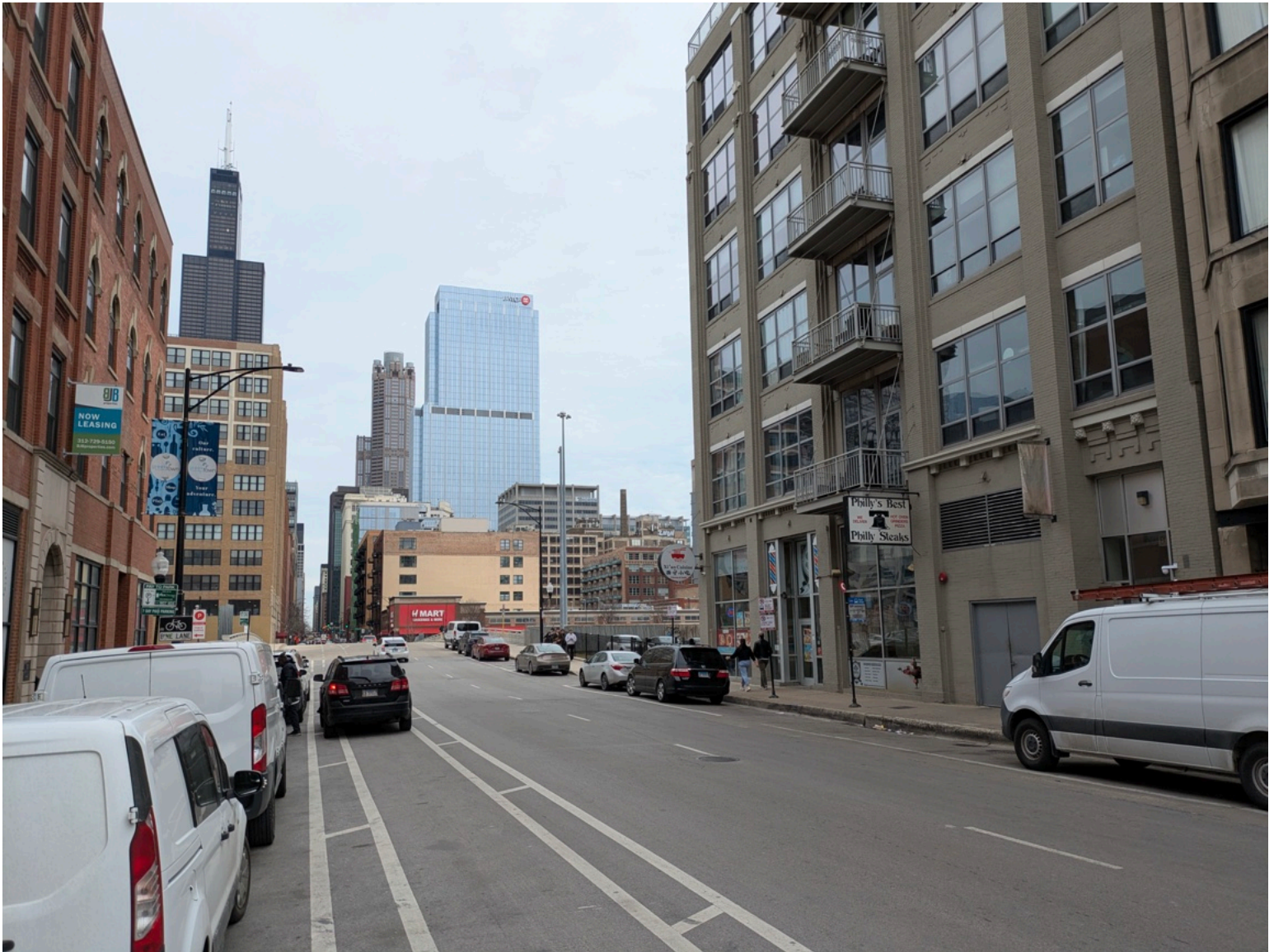
Present-day location of 166 W. Jackson (approximate location was on the right side of the street just past the building) Photo Credit: Michael E. Byczek. Copyright 2026.
