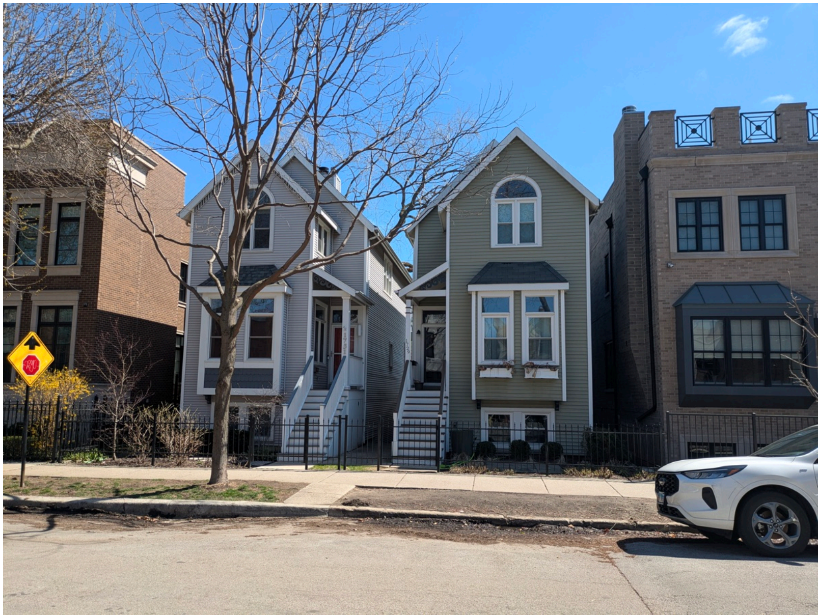
Present-day 1729 N. Wood (Wicker Park) [green house on the right] Original building was torn down Photo Credit: Michael E. Byczek. Copyright 2026.
