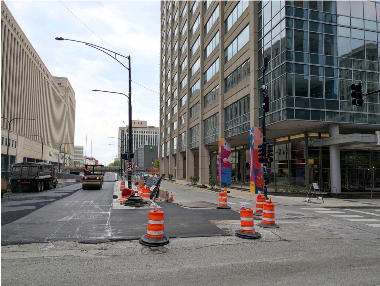
Present-day SW corner of Canal and Van Buren (looking south on Canal) Photo Credit: Michael E. Byczek. Copyright 2026.
