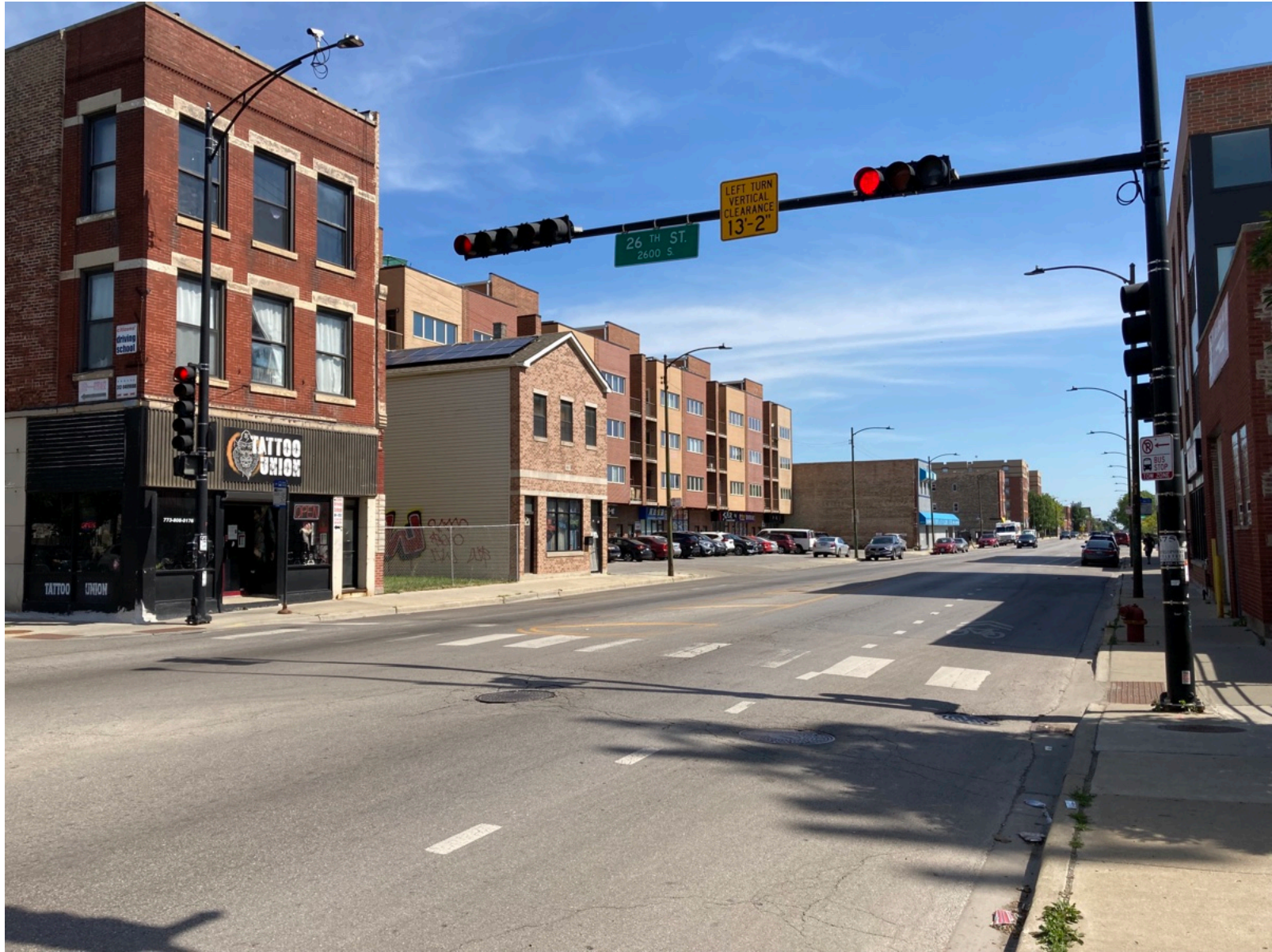
26th and Halsted (Bridgeport - Chicago, IL) Perspective from 26th and Halsted looking south on Halsted Photo Credit: Michael E. Byczek. Copyright 2022.
