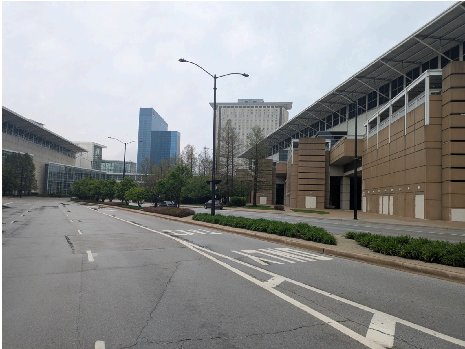
McCormick Place in the approximate location of the former intersection of 24th and Calumet Credit: Michael E. Byczek. Copyright 2026.
