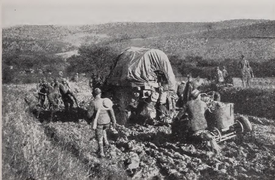
Engineers Working on Road Near Barricourt, November 4, 1918 Note condition of road
