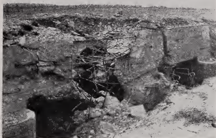
Effect of a Direct Hit on a German Concrete Shelter
