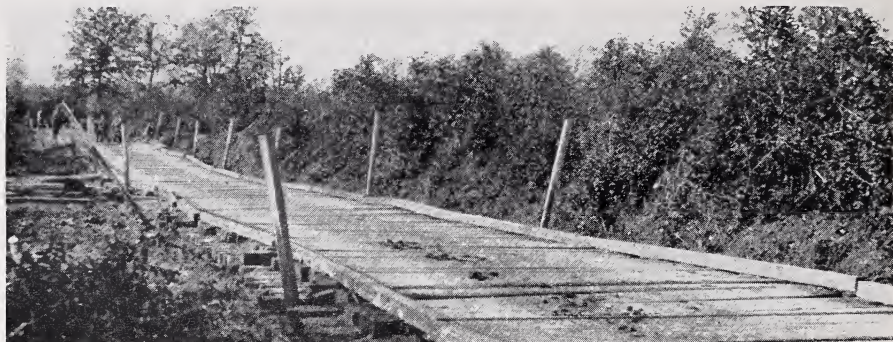
Section of Avocourt-Montfaucon Road Showing Plank Construction
