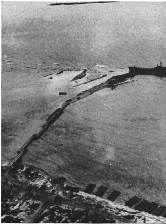
SEABEES AND ENGINEERS , working under fire, had this causeway fully operative by D-plus 6 to bridge the reef. Angaur Island in background.
